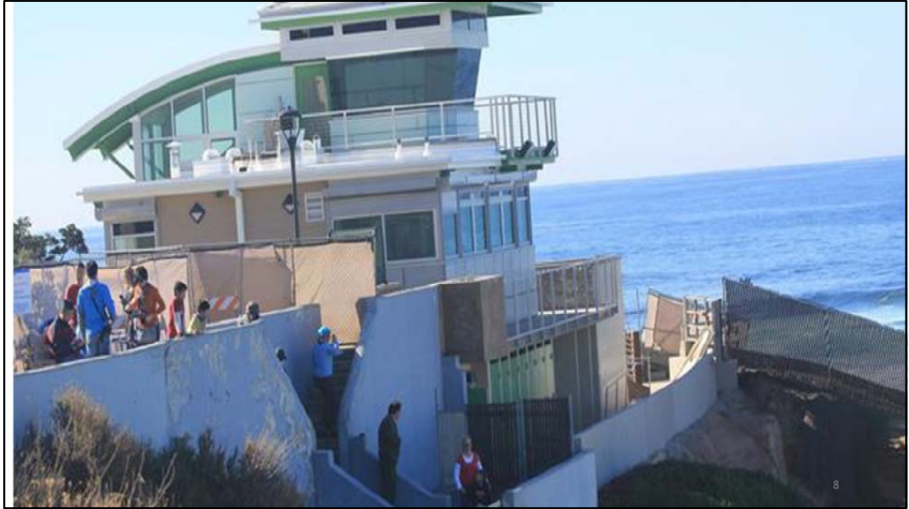
Lifeguard Station nearing completion.
