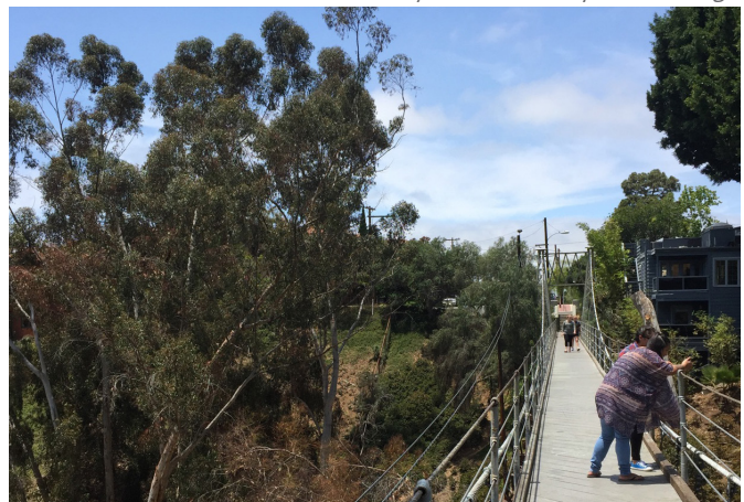
Spruce Street Suspension Bridge
