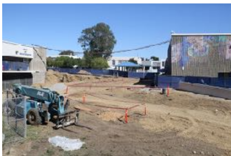
Construction at SDHS, LaBella Photography, 2023, SDHS Alumni
