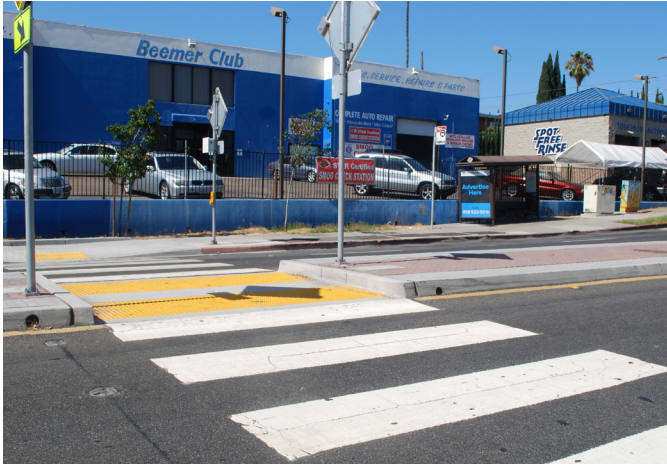
Mid-block crossings can be considered and utilized to accommodate pedestrian access across streets with infrequent intersections.
