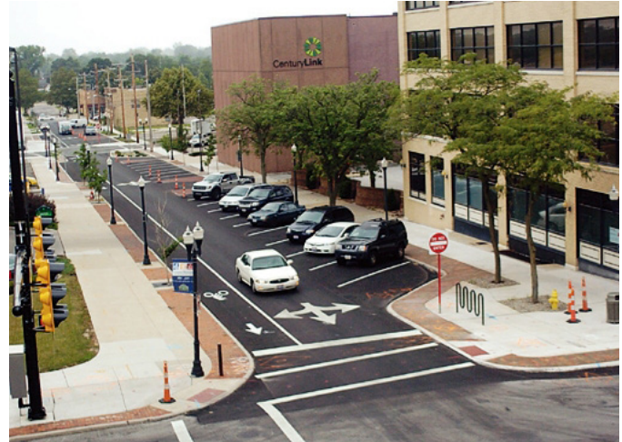
Reversed angled parking could provide opportunities for more parking in the community and safer streets.
