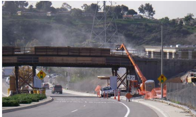
Sandblasting Photo. Source: WESTON, 2006.
