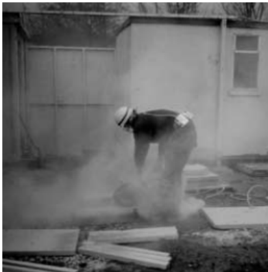
Concrete Cutting Photo Source: Health and Safety Executive (CIS No. 54)
