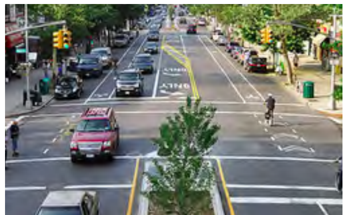
The Complete Streets concept encourages street connectivity and aims to establish a comprehensive, integrated mobility network for all modes of travel.
