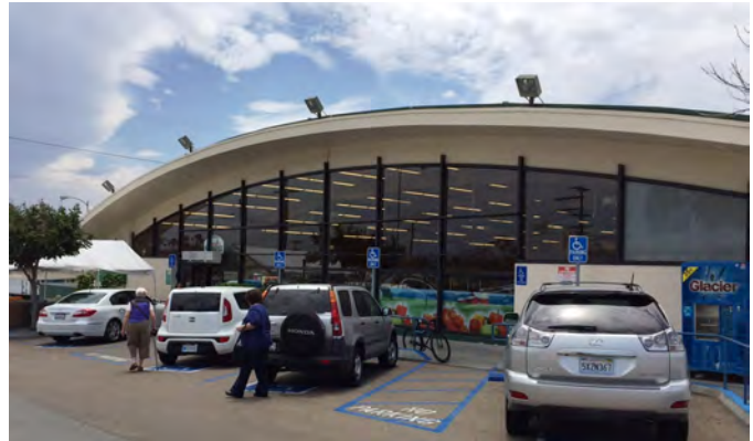
4175 Park Boulevard, an identified potentially significant individual resource in the community was built in 1965 represents the Googie architectural style.
