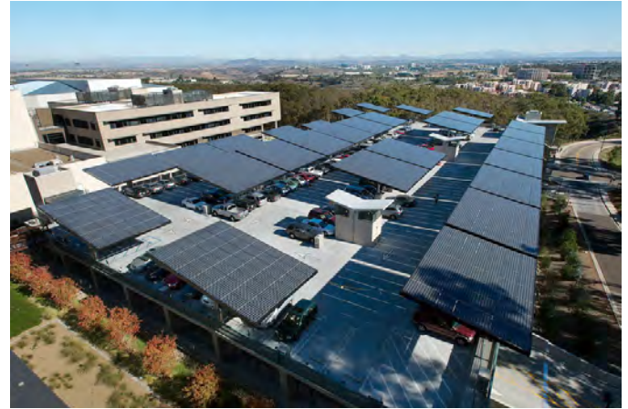
Opportunities exist for the installation of photo-voltaic systems atop the flat roofs of many businesses in North Park's business districts.
