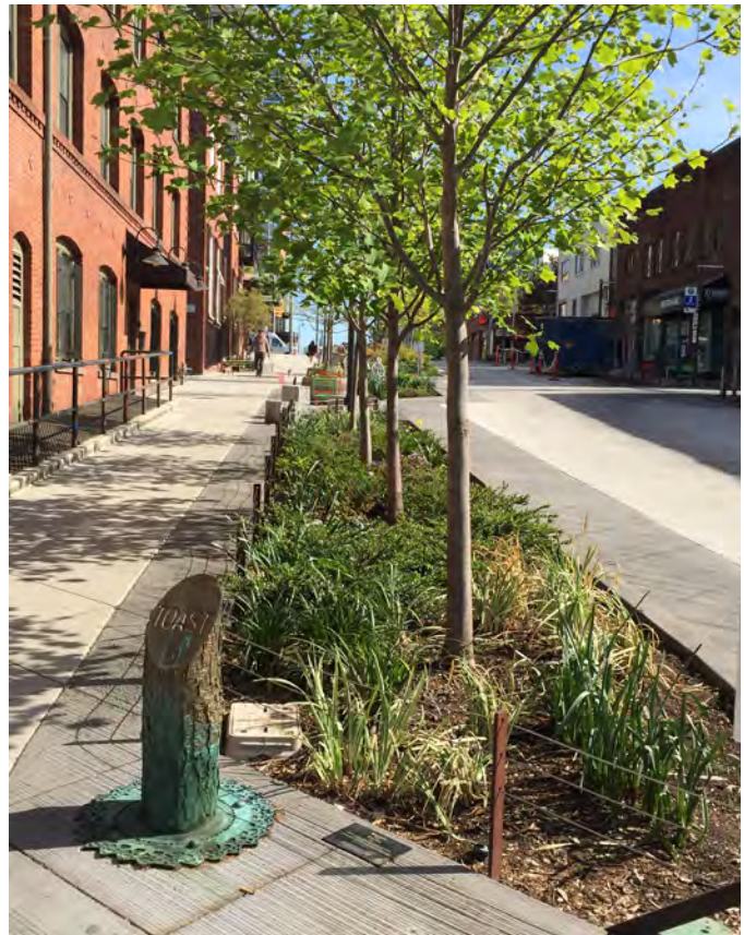
Bioswales and other filtering techniques can serve the dual function of creating aesthetically pleasing urban areas and treating stormwater.
