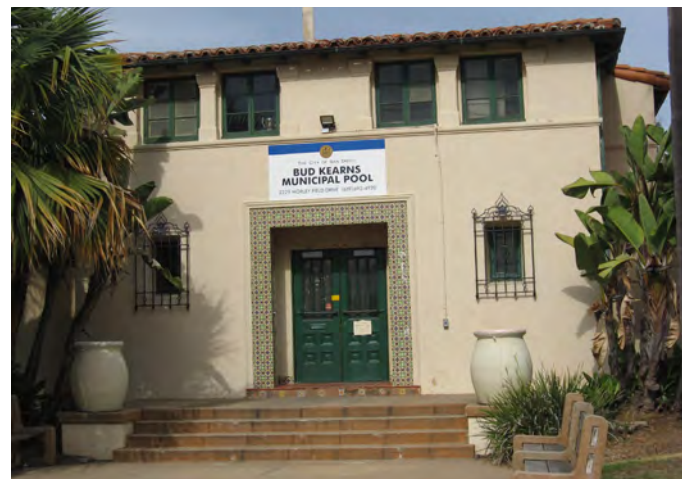
Bud Kerns Pool House, within Balboa Park, to be expanded to provide an aquatic complex for the North Park community.
