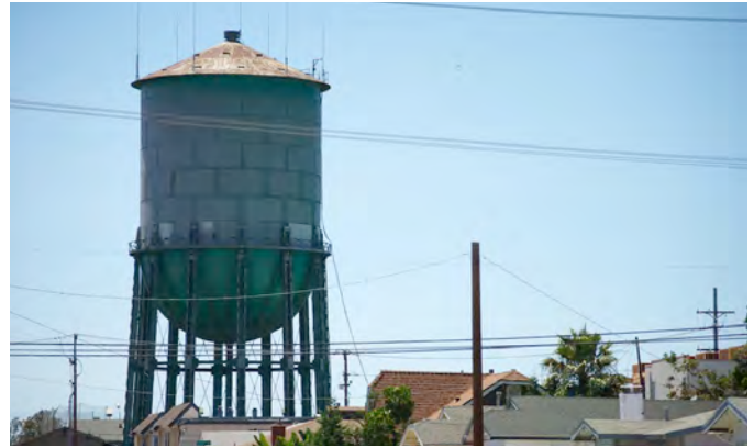
The University Heights Water Storage and Pumping Station Historic District is listed on the National Historic Register of Historic Places.
