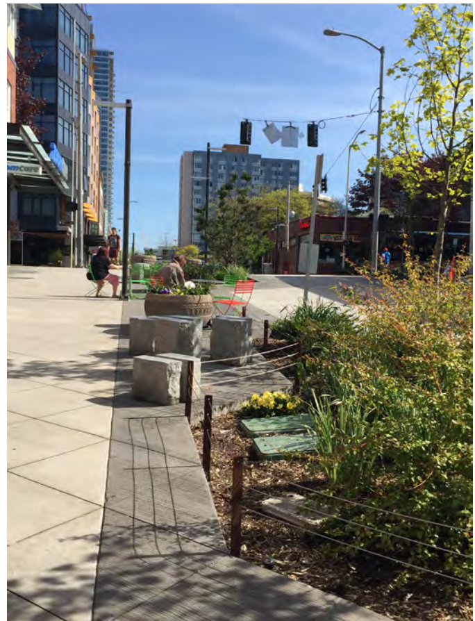
Bio-filtration techniques can work together with storm drain infrastructure to treat storm water and reduce storm water pollution.
