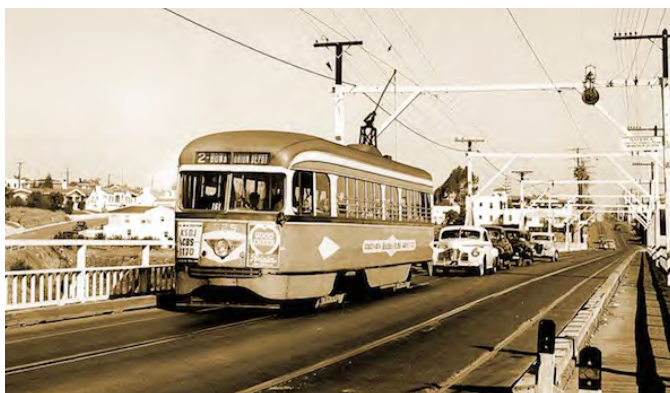
The image above shows the No. 2 trolley line crossing Switzer Canyon during the 1940s enroute to Golden Hill and eventually terminating at Broadway and Fifth Ave Downtown.
