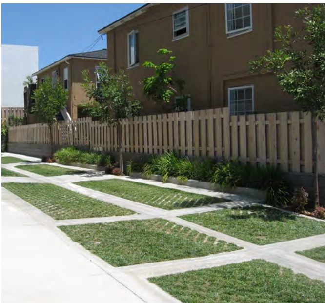
Residences can contribute to stormwater filtration efforts by reducing the amount of impervious driveway surfaces.
