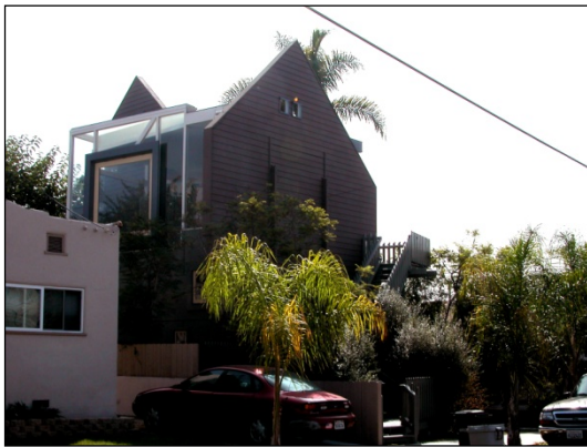
Figure B.57: Deconstructivist, c.1990. (4061 Randolph Street, 100604-76.)
