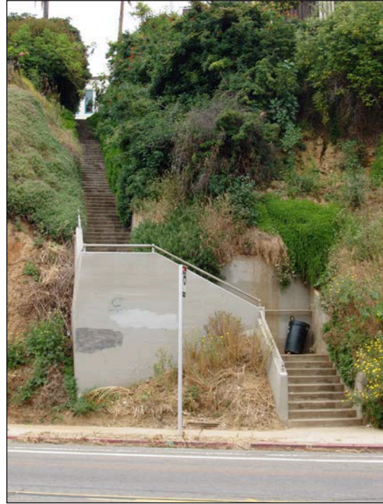
Figure F.34: Public Staircase, Upper Reynard Canyon.
