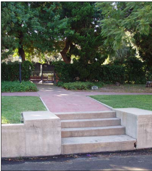
Figure F.19: Retaining Wall/Stairs at Street.
