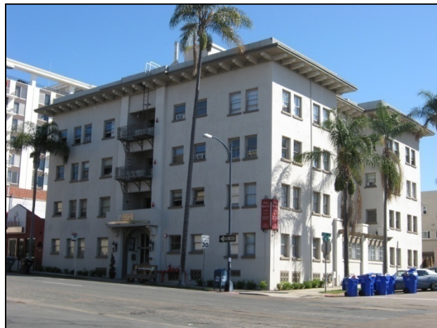
Figure 14. Kirkland Apartments, 2309 5 th Avenue, HRB #483 Source: Planning Department Staff
