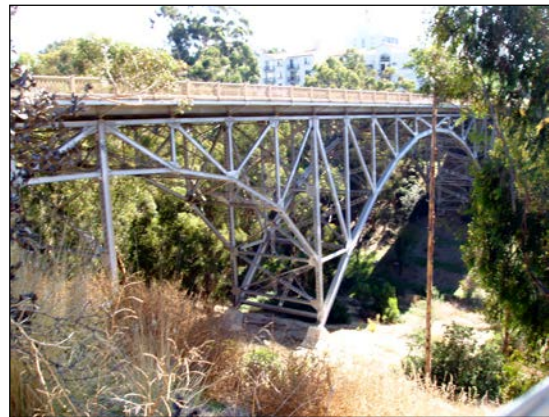
Figure F.25: First Avenue Bridge, 1993.
