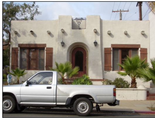
Figure B.33: Pueblo Revival, 1925. (418 Walnut Avenue, 110805-16.)
