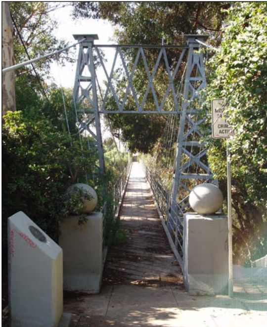
Figure F.23: Spruce Street Suspension Bridge, 1977.
