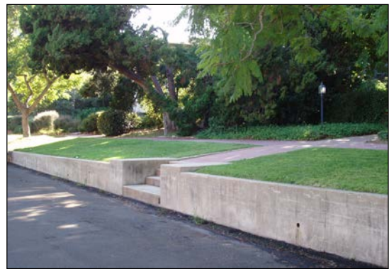
Figure F.39: Seventh Avenue retaining wall at roadbed, Hillcrest, Crittenden's Addition.
