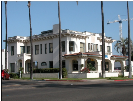
Figure B.23: Italian Renaissance Revival, 1911. (2900 6 th Avenue, 081004-01.)
