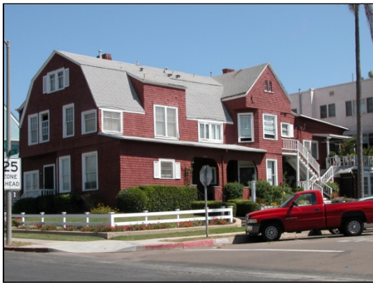
Figure B.8: Shingle with Dutch Gambrel Roof, c.1900. (114 Kalmia Street, 090805-29.)
