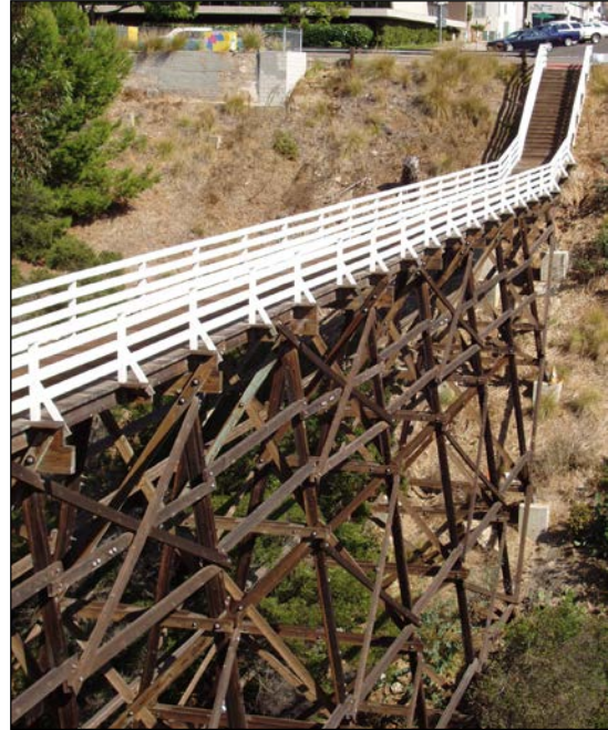
Figure F.24: Quince Street Bridge, 1987.
