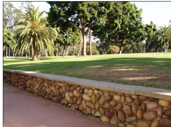
Figure F.40: Balboa Park Cobble Wall, Upas St./Sixth Avenue, Hillcrest
