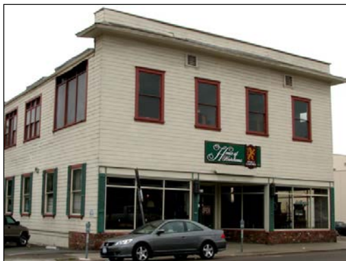
Figure B.12: Victorian Wooden False Front, 1905. (801 University Avenue, 081604-40.)
