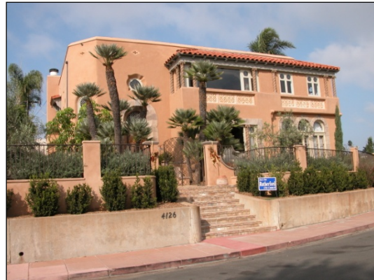
Figure B.4: Moorish Revival, c.1925. (4126 Arden Way, 102605-32.)
