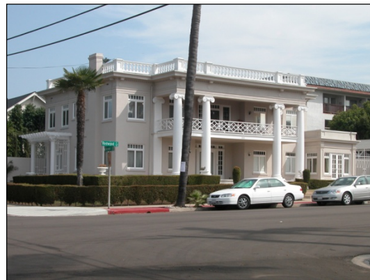
Figure B.16: Neoclassical, c.1910. (202 Redwood Street, 092105-40.)
