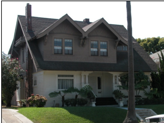
Figure B.34: Arts and Crafts, 1912. Architect Thomas Harbo Rynning. (1871 Sunset Blvd., 101905-83.)
