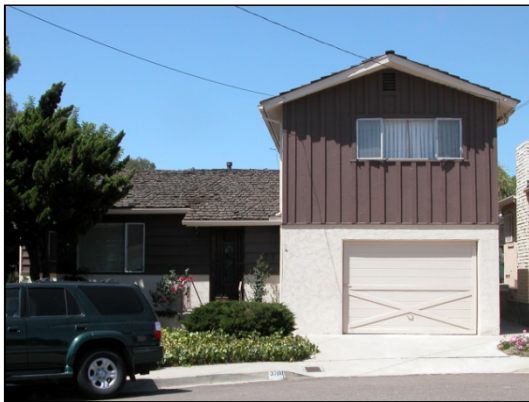
Figure B.54: Split Level, 1958. (3708 Hawk Street, 090204-03.)
