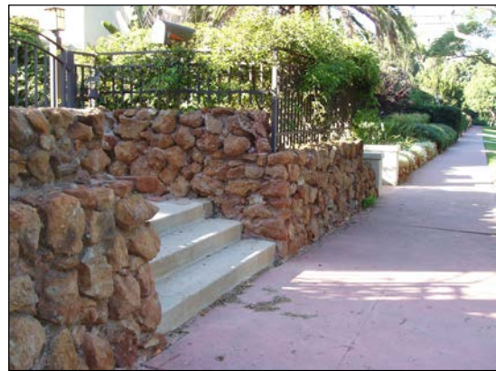
Figure F.21: Red Sandstone Front Yard Walls.
