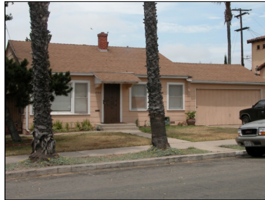
Figure B.51: Minimal Traditional, 1943. (4142 Maryland Street, 070704-66.)
