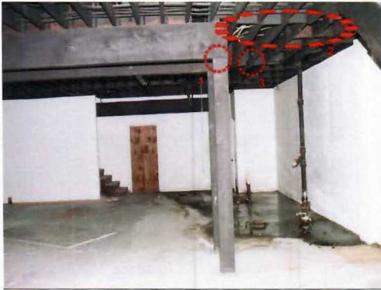
Image #5 show the portion of the floor with out any support at the middle with spliced joist
