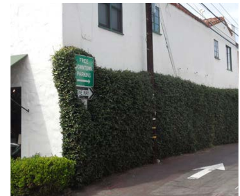
Improve alley aesthetics with landscaping, wayfinding, specialty paving, public art, and lighting
