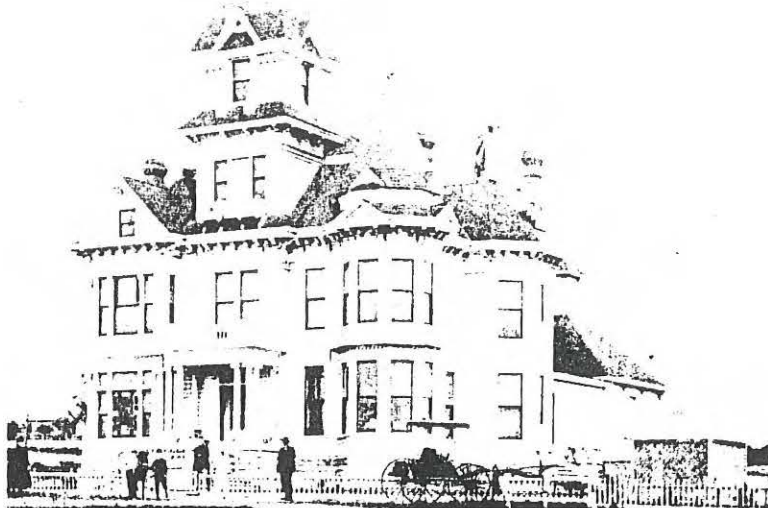
Matthew Sherman's home (now apartments), in 1890; photo from Title Insurance & Trust Historical Collection.
