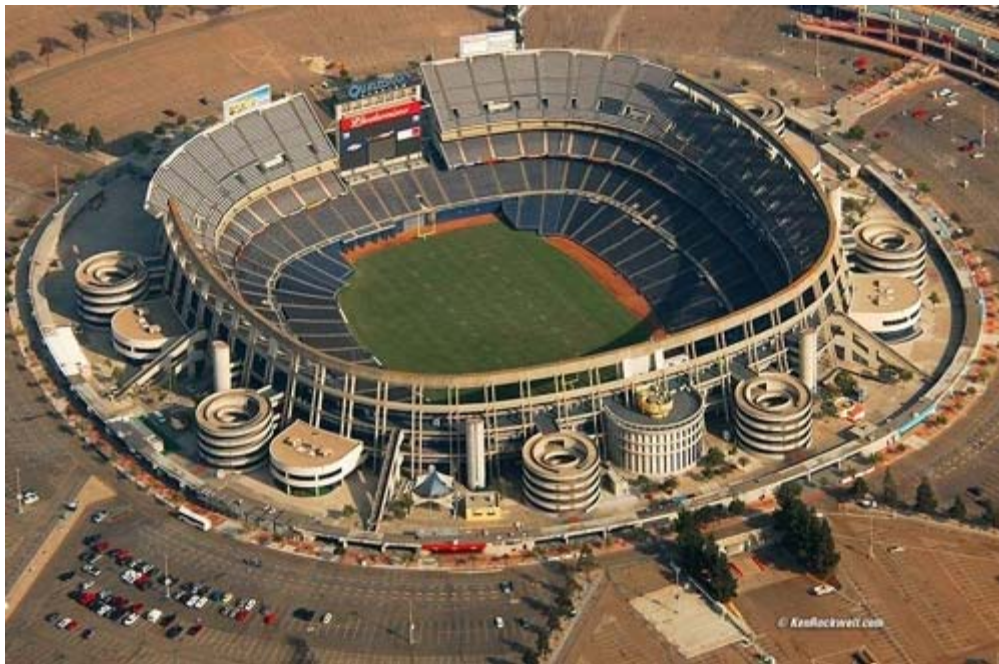
Figure 1 Aerial View of Qualcomm Stadium
