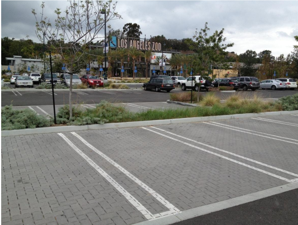
Figure 4. Permeable pavement and bioswales at the Los Angeles Zoo and Botanical Gardens (source: Tetra Tech, Inc.)
