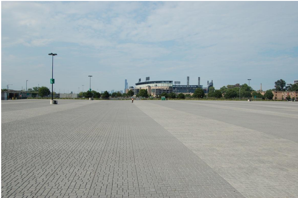
Figure 5. Mechanically-installed permeable pavement at US Cellular Field in Chicago, IL (source: North Carolina State University – Biological and Agricultural Engineering)
