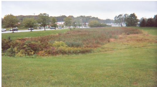
Figure 1. Example of a Dry Extended Detention Basin
