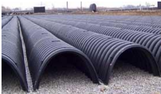
Figure 1. Example of a Subsurface Infiltration Gallery
