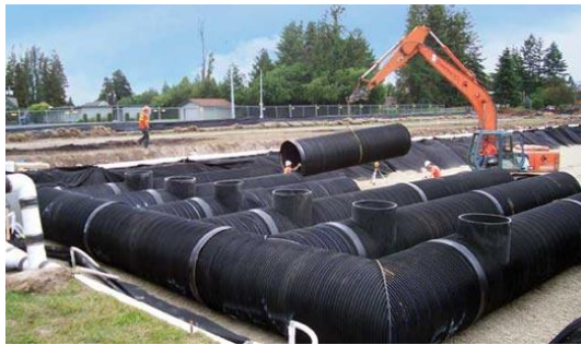
Figure 1. Example of a Subsurface Detention Gallery
