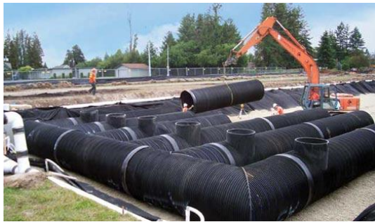
Figure 1. Example of a Subsurface Detention Gallery
