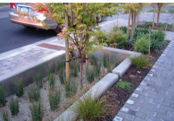
Eco-roofs, permeable paving, and bioswales are strategies to reduce solar heat gain and integrate stormwater management.
