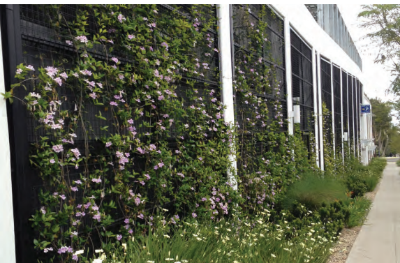
Wrap parking with active building uses (top). Consolidate parking entrances and minimize visual impact (middle). Use vines, shrubs, and trees to screen parking (bottom).
