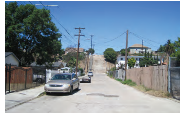
Parts of Southeastern San Diego, especially along Chollas Creek, have steep slopes that can present a hazard if the slope becomes unstable due to earthquakes, extensive rainfall, or excavation.
