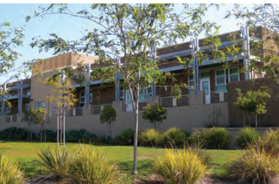
Sherman Heights Community Center, the Logan Heights Library, and the Educational Cultural Complex serve residents of Southeastern San Diego.
