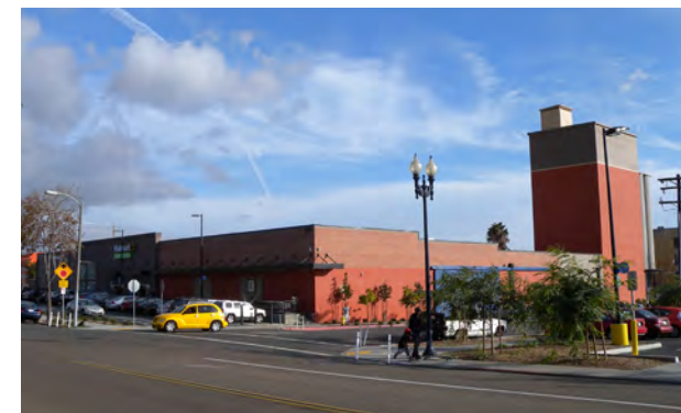
Sherman Heights Community Center (top), Bread & Salt (the former Weber's Bakery, middle), and Walmart Neighborhood Market (the old Farmers' Market Building, bottom) are examples of rehabilitation and adaptive reuse.
