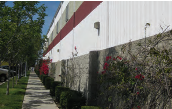
The Comm22 development contributes to an active mixed use “village” (top). In industrial areas, exterior wall materials that contain integral colors and textures are encouraged (bottom).
