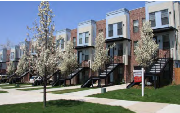
An extension of Alpha Street would become the spine of a new mixed-use neighborhood integrated with surrounding residential areas.
