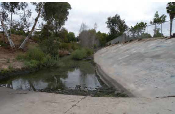
Stormwater swales and permeable paving (top and middle) allow water to infiltrate, preventing polluted runoff from entering streams (bottom).
